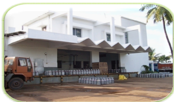
Front View of the Tirtol Dairy
