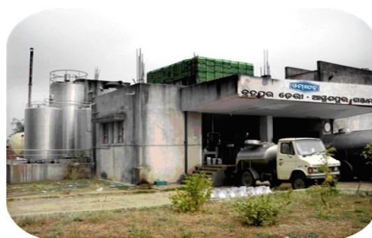
Front View of the Berhampur Dairy
